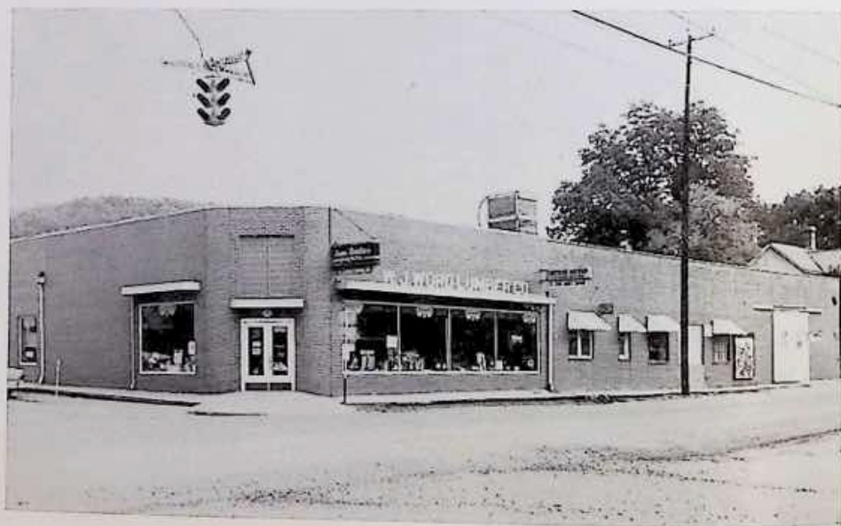
MAIN STORE BUILDING
